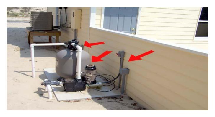
The above picture illustrates violations of **Section AG105.4 – Prohibited Locations**. The placement of this pool equipment and supporting electrical wiring help aid in climbing the barrier.
