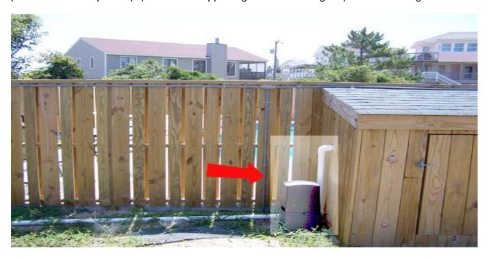
This barrier is 5 feet high and the lowest part of the pool equipment shed is 4 feet high. The horizontal members are spaced less than 45 inches apart so the verticals are spaced no more than 1 ¾ inches and the electrical conduit is OK. Problems: the optical lighting unit and the plumbing pipe location assist in climbing the barrier.
