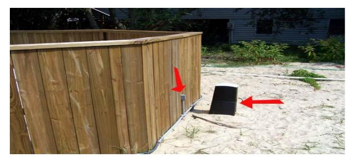
This barrier meets the minimum 4 feet height and barrier wall construction requirements but the location of the optical lighting equipment and the electrical device box provide assistance in climbing the barrier thus violating the provisions of **Section AG105.4 Prohibited Locations**
